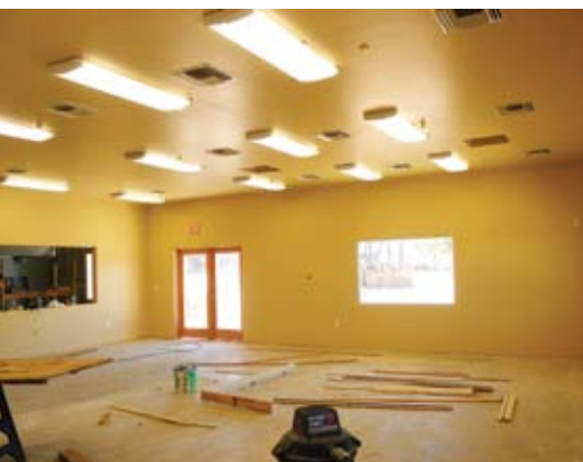
The new Chapel starts to take shape.
